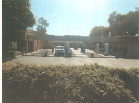
Photo #2: The study site fueling area
